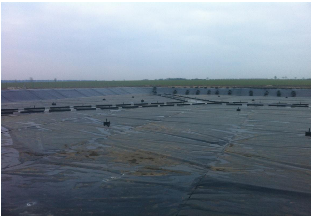
Figure 4. Lagoon fitted with floating cover.
